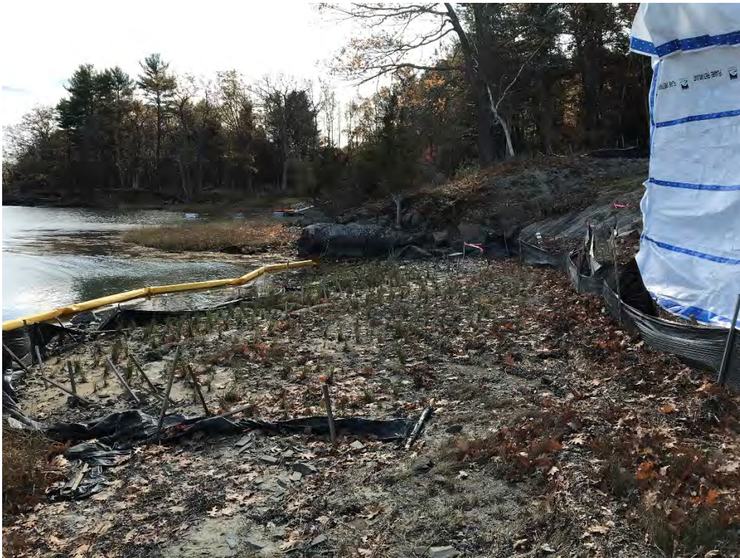
Fig 2: Toe of the slope and salt marsh restoration at the Eversource property/west side of the bay. Viewing south. (11-03-20)
