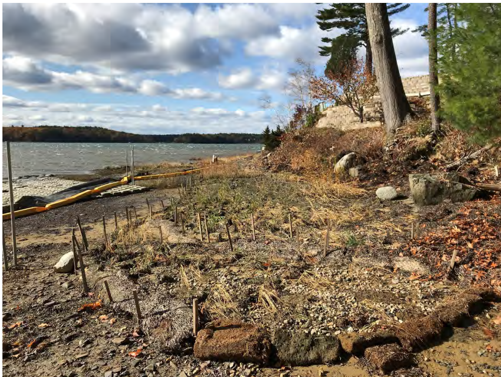
Fig 6: Salt marsh restoration at Gundalow Landing/east side of the bay. Viewing northwest. (11-03-20)
