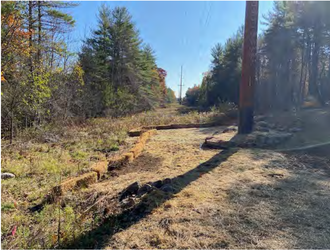
Fig 7: Str. 89 work area graded and mulched with straw. Viewing southeast. (11-04-20)
