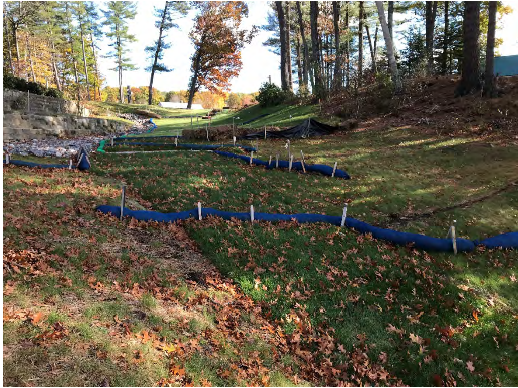
Fig 4: Slope below the manhole at Gundalow Landing/east side of the bay. Viewing east. (11-03-20)
